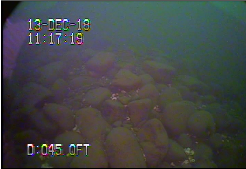
Figure 6 Rock below SB 10-12 End Sill.
